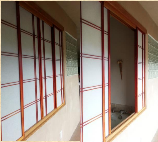
Shoji screens aide in bathroom ventilation
