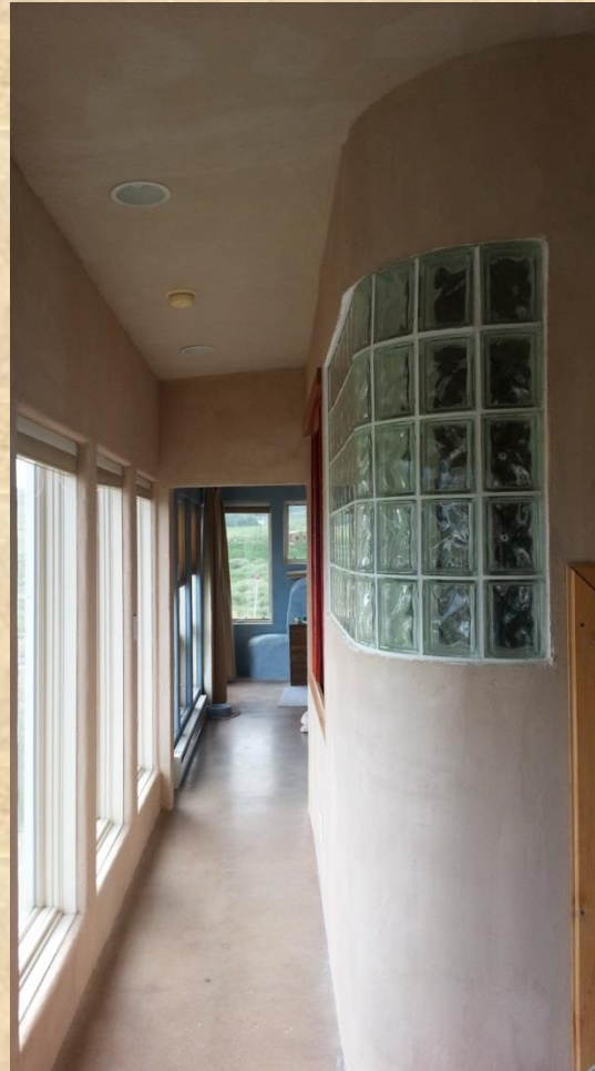
Curved, partial glass block walls on bathrooms provide light into spaces without using electricity
